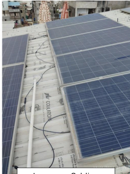
Improper Cabling
